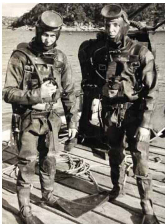
Photo 20. Commando divers in Sydney in early 1960's with Compressed Air Breathing Apparatus (CABA) with Porpoise 2 nd Stage demand valves and first-generation wet suits. Source. ACA Vic Historical Collection
