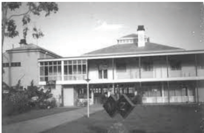
Post-war photograph of the ZES main building Source:
